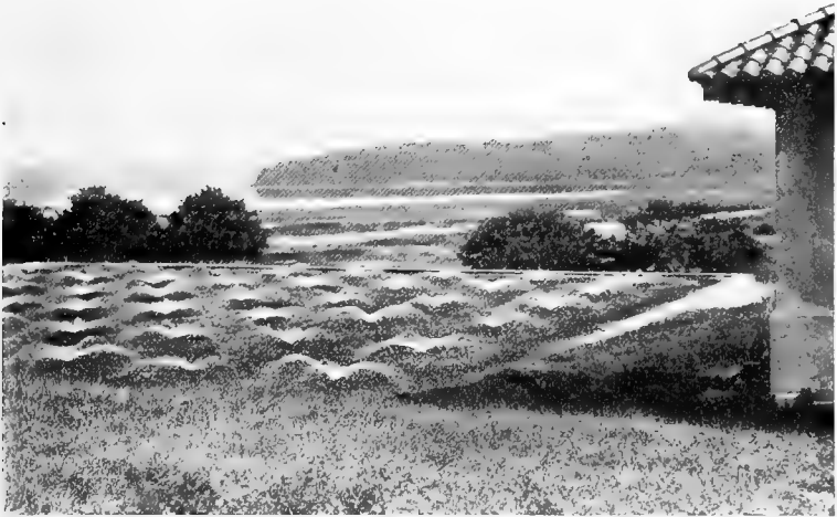
Fig. 46.—Sprinkling sewage over the stone bed of a sewage disposal plant.
